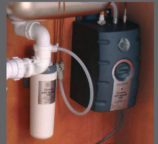
The hot water boiler and initial filter are included with the tap.
